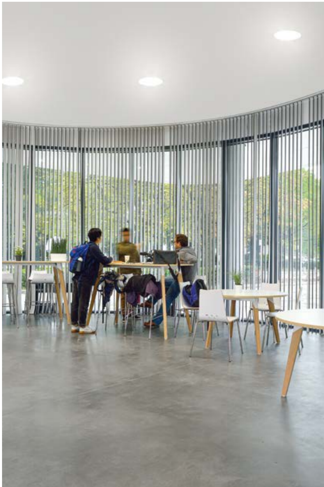
Acoustic blinds in front of glazing. The Centre for Creation and Innovation (MaCI) of the University of Grenoble Alpes in Saint-Martin-d'Hères, east of Grenoble. Architects: Jacques Ripault Architecture, 2019.
